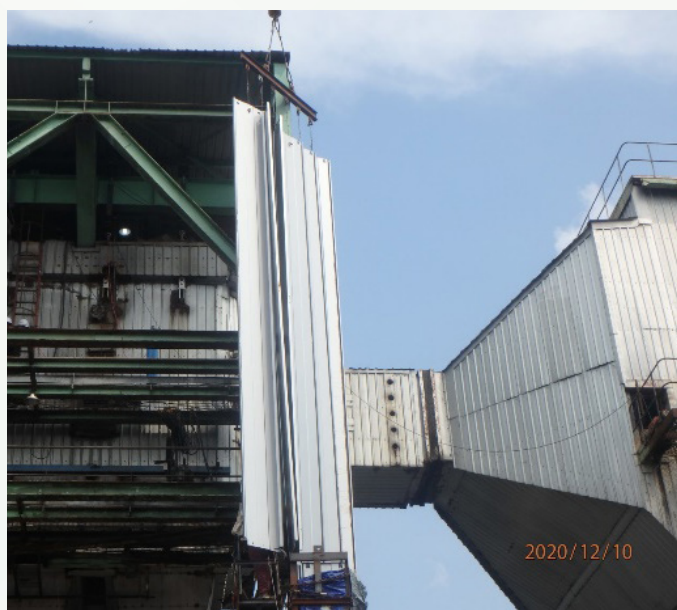
Lifting process of CE
