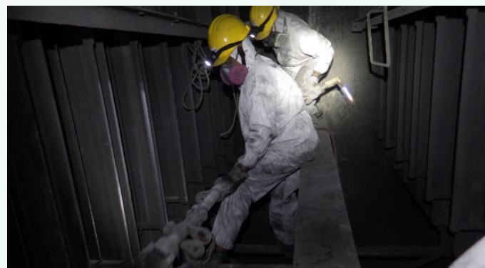
ESP inspection and maintenance
