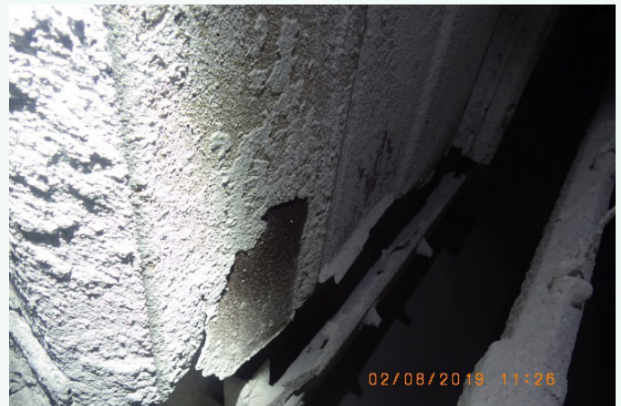
Severely corroded CE
