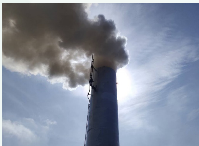
Black smoke coming out of the stack indicating high emission and opacity
