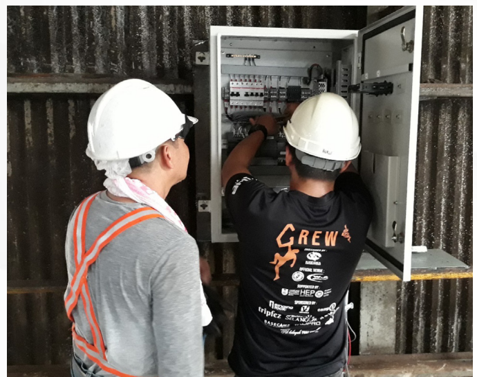
ABS working with the mill team to Implement a Control Panel with Edge Device & 3G Gateways to support IoT's in a clients mill
